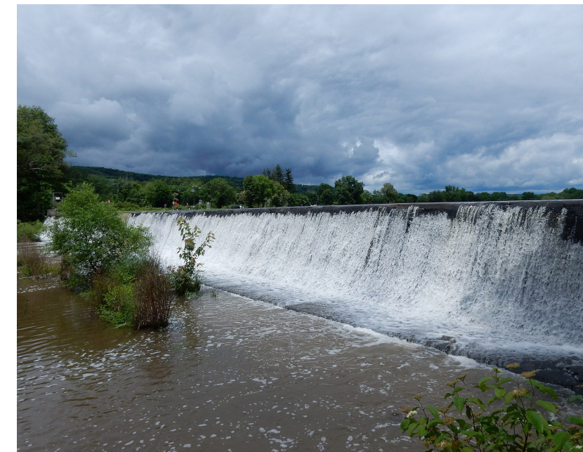
Deer Lake Dam in Schuylkill County
